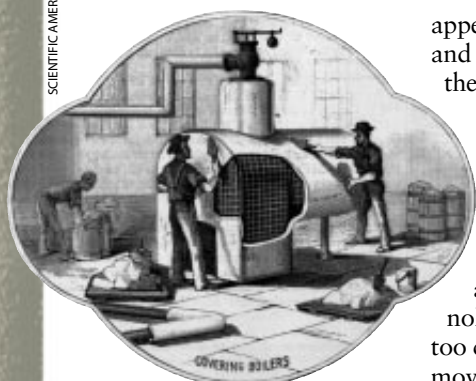
Asbestos used as insulating material
