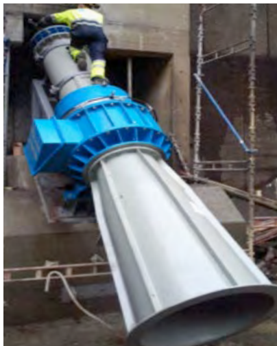
Source: Opsahl 2013 Figure 1-11. Inclined (left) and horizontal (right) integrated turbine-generator technology installed without a powerhouse
