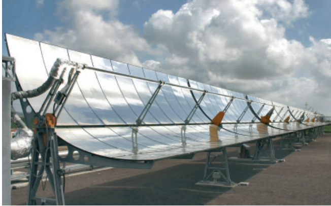
Figure 1 – CSP Parabolic Trough Solar Collectors
