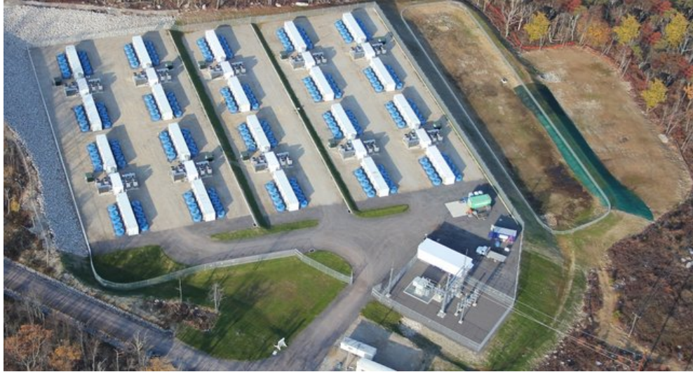
The flywheels are buried in the ground to reduce visual impact and run silently
