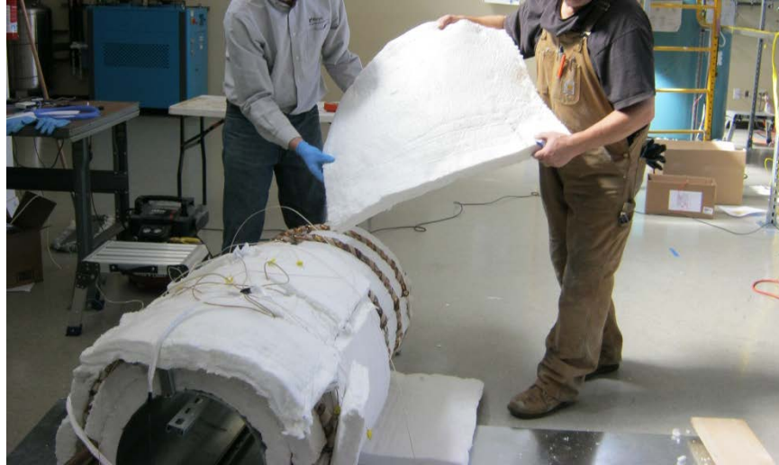
Figure 39. Insulation is then added to the exterior followed by a sheet metal casing, as was shown for the interior in Figure 11 (exterior sheet metal is not shown).
