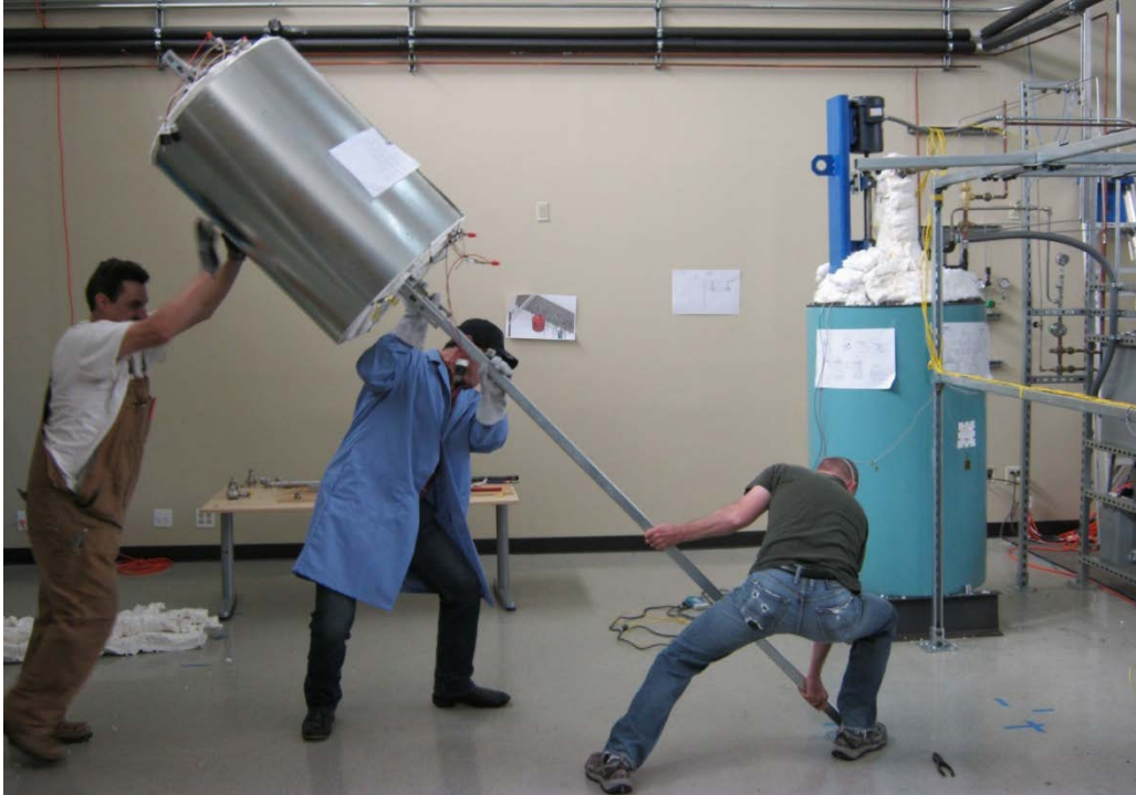
Figure 33. FX encased in a stainless steel jacket, being installed in the system.
