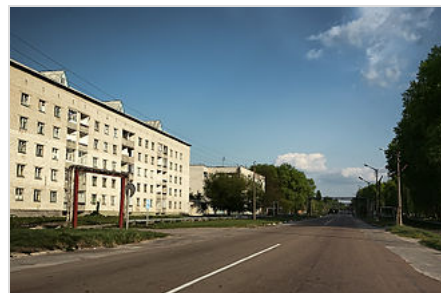
Abandoned buildings in Chernobyl
