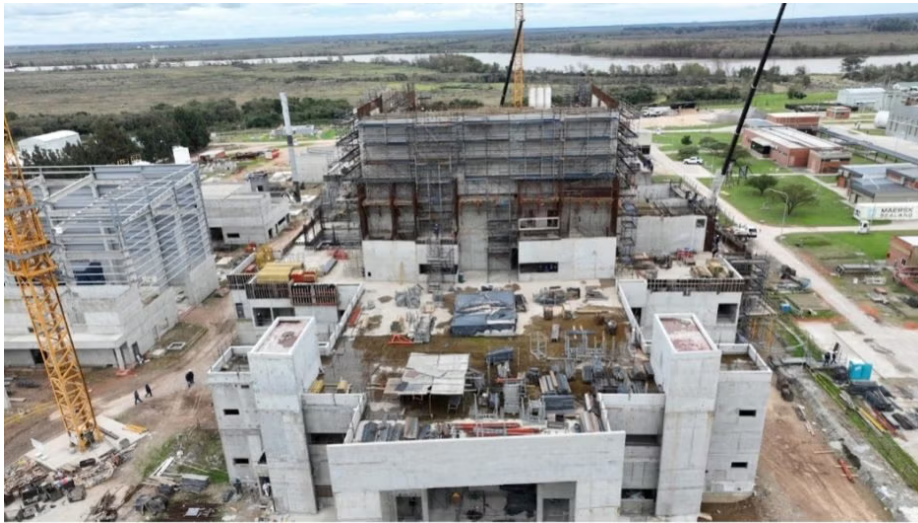
The CAREM-25 SMR construction site in August 2024 (Source: CNEA)
