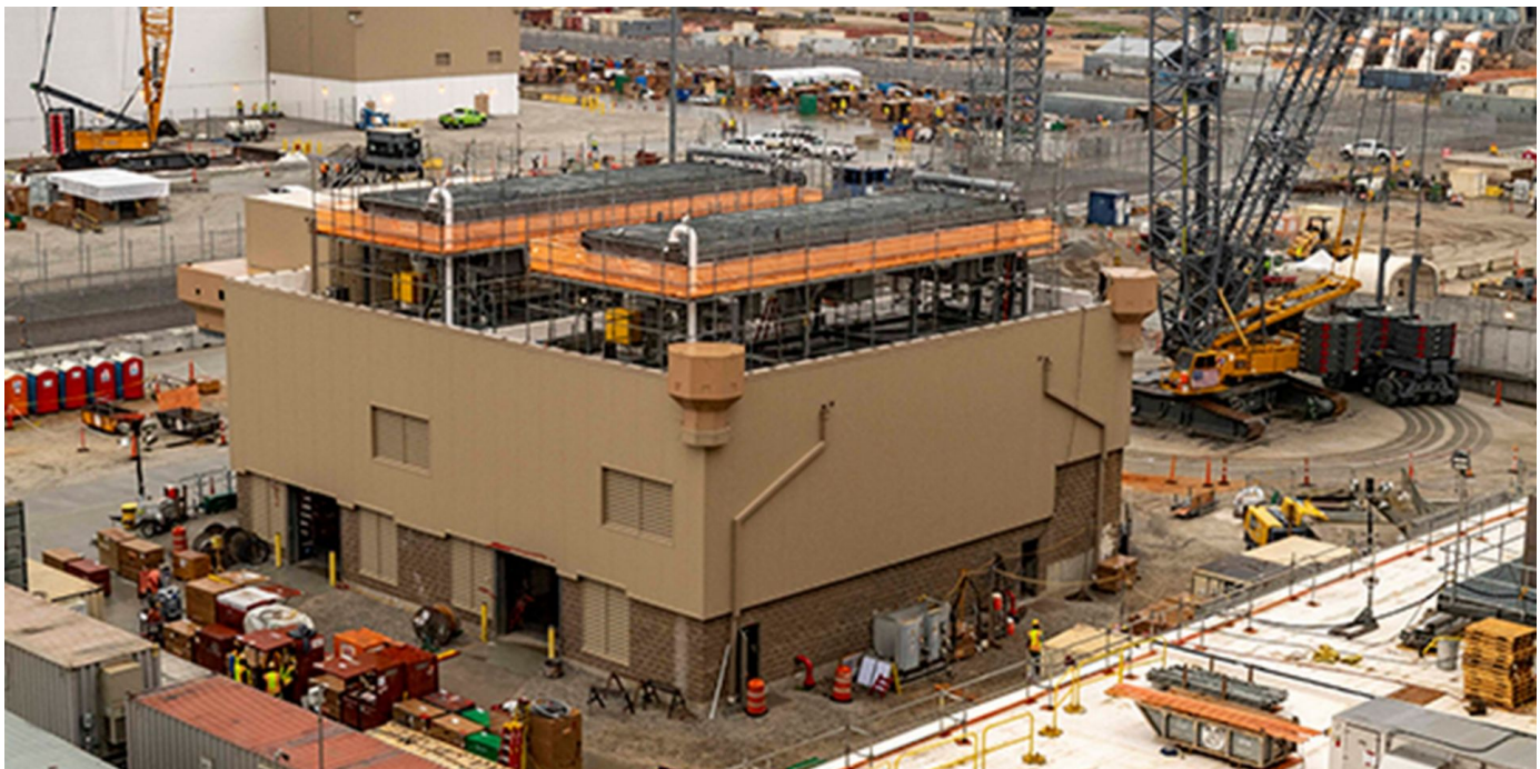
The Vogtle-4 diesel generator building in March. (Photo: Georgia Power)
