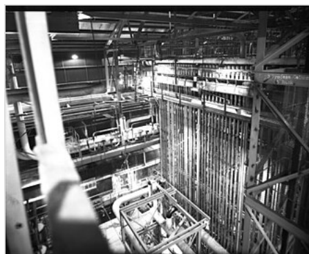
Another view of the columns
