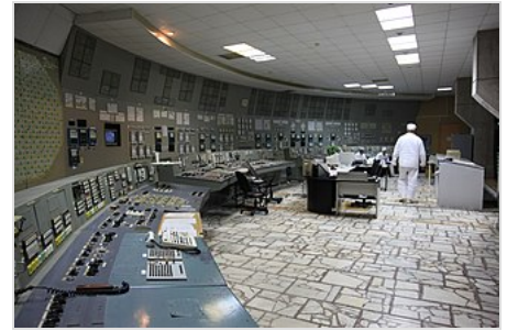
The control room of Chernobyl Unit 3, a second generation RBMK. A large circular mimic display for every channel or core map is on the left
