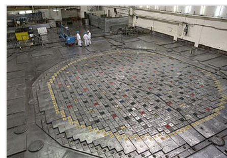
RBMK reactor with fuel channel covers
