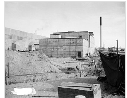
The 224-T plant under construction, showing the transfer pipes
