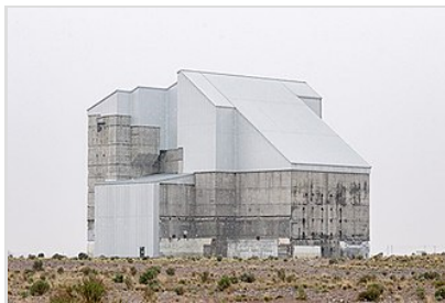
H Reactor after cocooning
