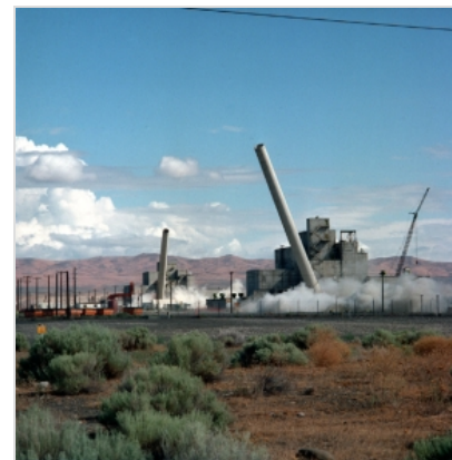
Decommissioning D Reactor
