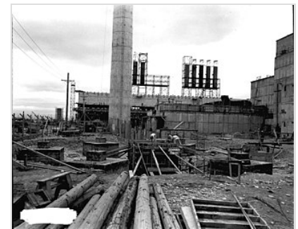
B Reactor construction (1944)
