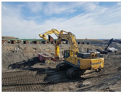
Heavy equipment removing buried pieces of pipe filled with contaminated waste
