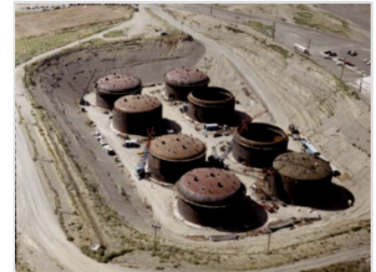
Hanford storage tanks in 2014
