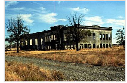
Hanford High School after abandonment
