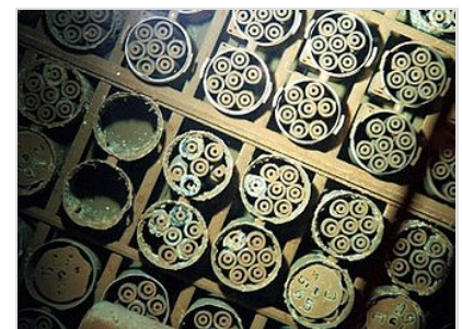
Spent nuclear fuel stored underwater and uncapped in Hanford's K-East Basin
