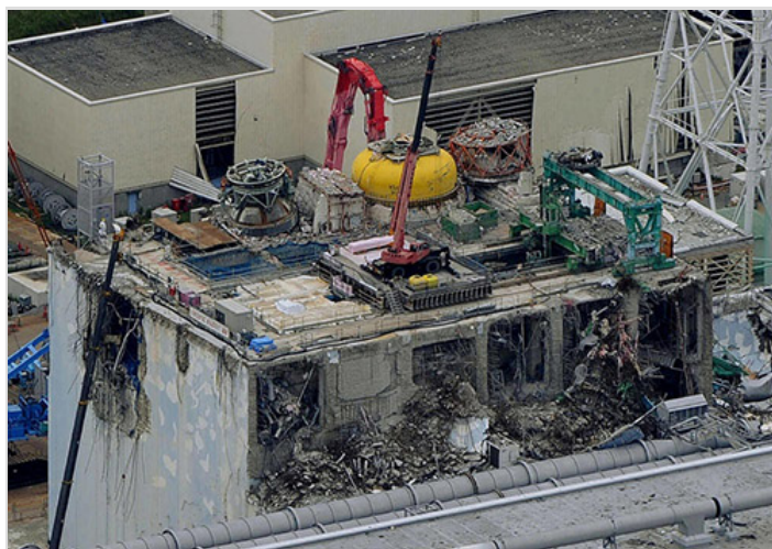
The unit 4 reactor building after the explosion. The yellow object is the reactor's removed PCV head. The removed black RPV head with its lifting frame attached is to the left. Both had been removed to allow refueling at the time. The green gantry crane carries fuel between the RPV and the spent fuel pool.
