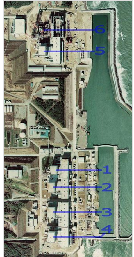
Aerial view of the station in 1975, showing separation between units 5 and 6, and 1–4. Unit 6, completed in 1979, is seen under construction.
