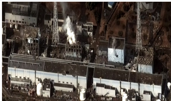
The four damaged reactor buildings (from left: Units 4, 3, 2, and 1) on 16 March 2011. Hydrogen-air explosions in Units 1, 3, and 4 caused structural damage. [1]
