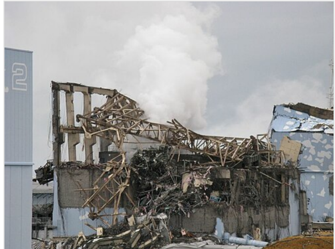
Unit 3 after the explosion on 15 March 2011.
