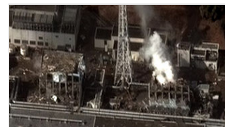
Three of the reactors at Fukushima Daiichi overheated, causing meltdowns that eventually led to explosions, which released large amounts of radioactive material into the air. [46]
