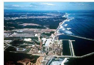
Plant still under construction circa 1971
