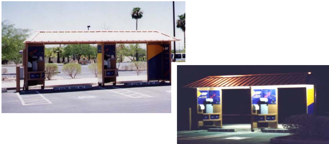
Figure 5-10. Level 2 public charge station with shelter, lighting, access control, and a customer service speaker phone incorporated.
