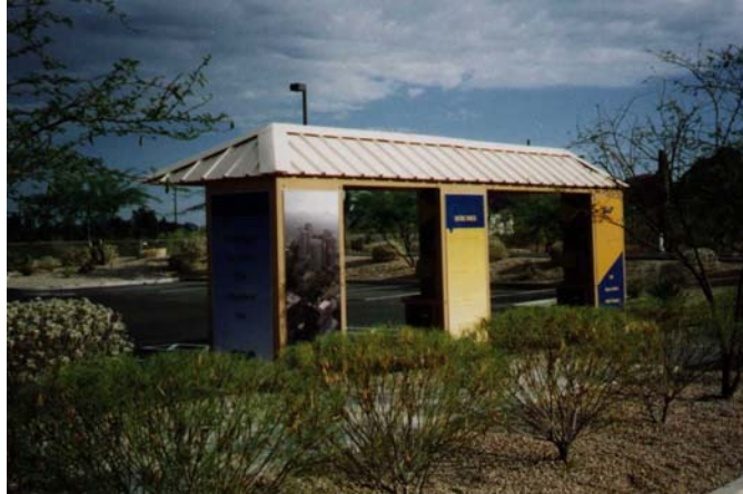
Figure 5-18. Public charging station with informational graphic panels.
