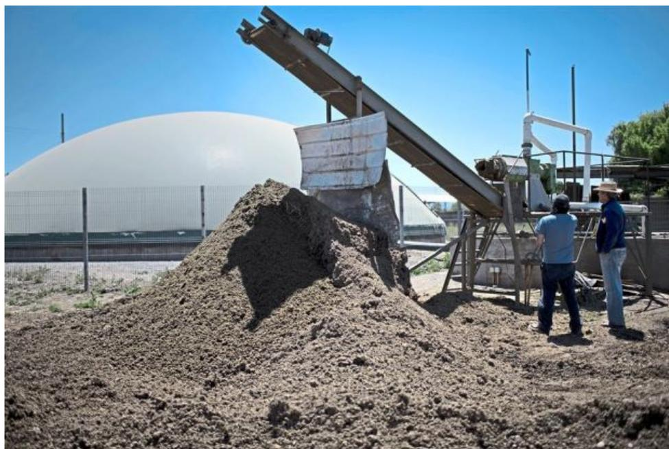
No wastes: The fermentation of pig and cattle manure generates organic fertiliser and biogas (for electricity generation). This biogas plant about 150km south of Santiago, Chile, generates up to 4MW of electricity for the farm's own use. — Photos by AFP
