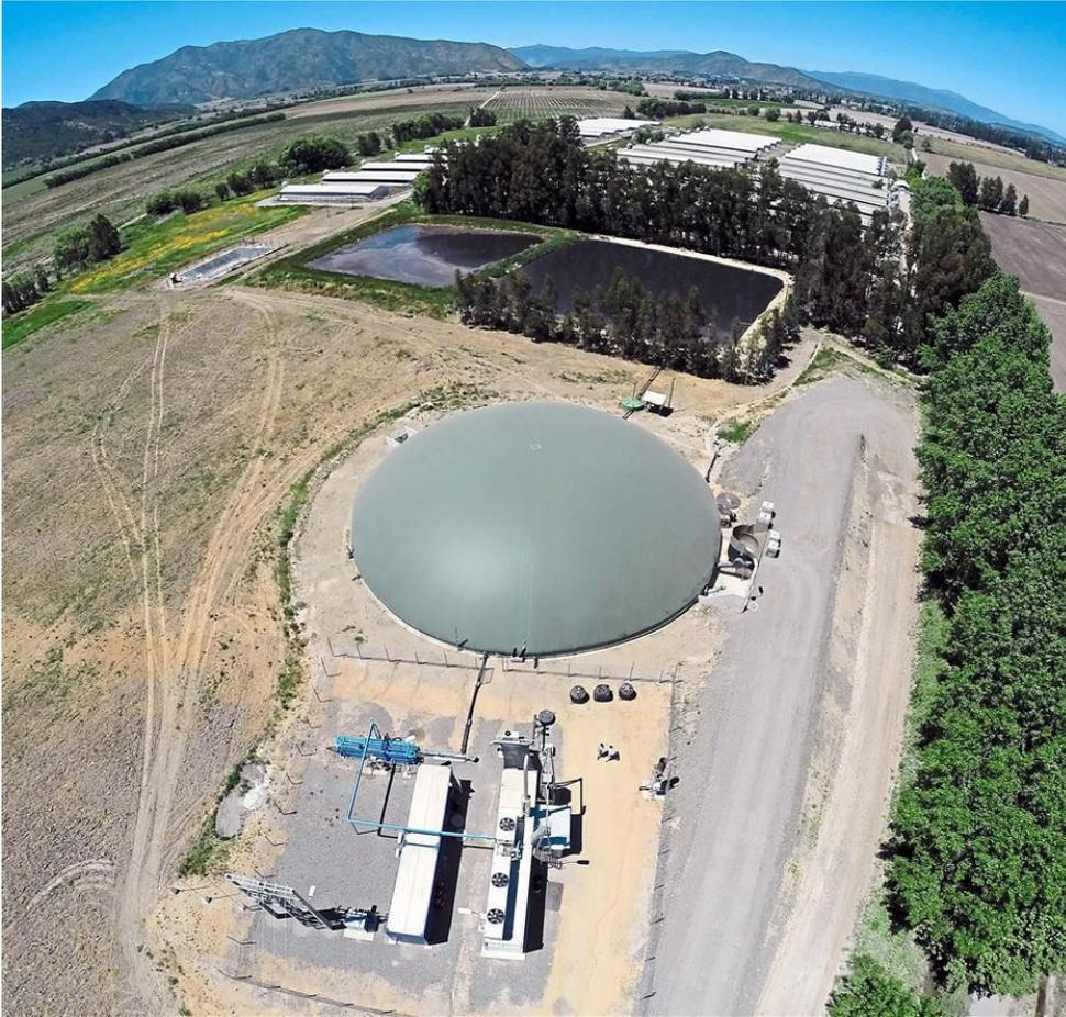
In this biogas plant about 180km south of Santiago, Chile, pig and cattle manure is decomposed in a digester to produce biogas (a mix of methane and carbon dioxide) that is then used to generate enough electricity to supply 2,500 homes.
