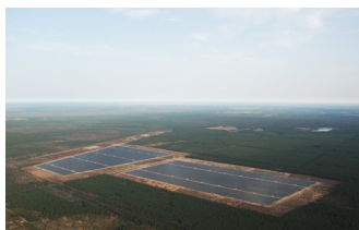
Lieberose Photovoltaic Park
