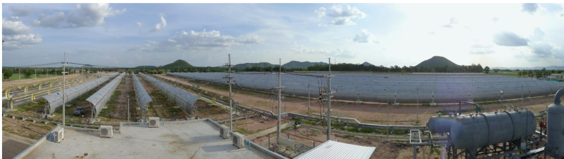
Figure 58: Kanchanaburi Solar Thermal Power Plant (source: Solarlite)
