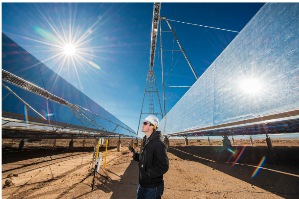
Steve Sellers of AREVA Solar stands amid the Compact Linear Fresnel Reflectors, the mirrors that focus sunlight to the top of the structure where molten salt is flowing. The resulting heat is stored and used later when the sun is not shining. Credit: Randy Montoya.
