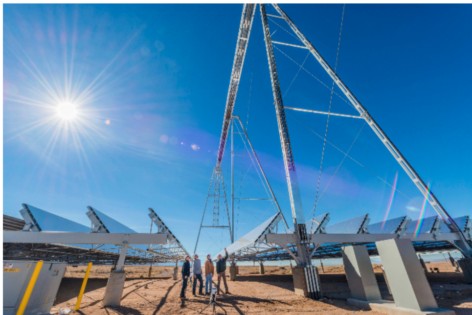
A team of Sandia National Laboratories and AREVA engineers examine the focal point of the sunlight reflected from the rows of mirrors on the ground. Credit: Randy Montoya.
