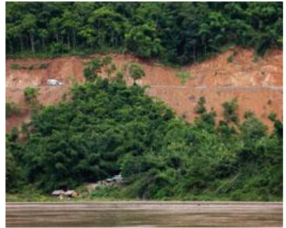
Road construction near the Xayaburi dam site. El Ali/Focus/eyevine
