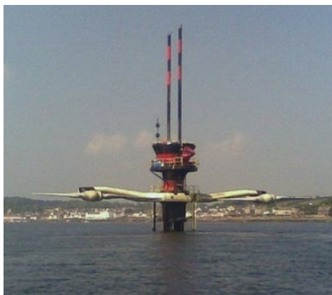
The SeaGen rotors can be raised above the surface for maintenance.
