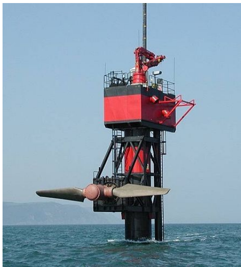
SeaGen's predecessor, the 300 kW 'SeaFlow' turbine off the north coast of Devon
