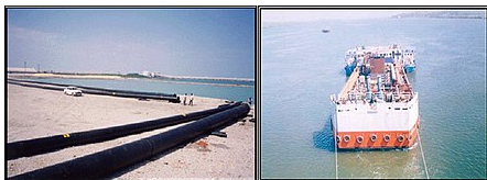
India – pipes used for OTEC (left) and floating OTEC plant constructed in 2000 (right)
