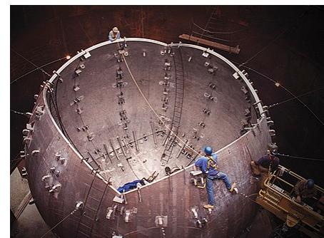
The NIF target chamber was so large it had to be built in sections.
