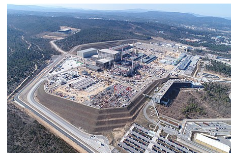
Aerial view of the ITER site in 2018
