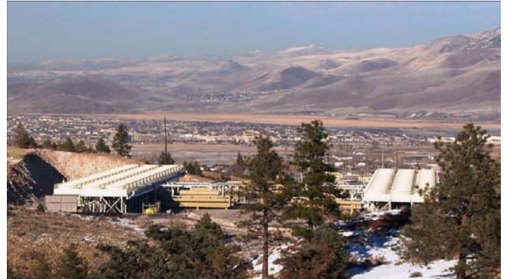
Figure 10: Burdett, NV, Binary Power Plant
