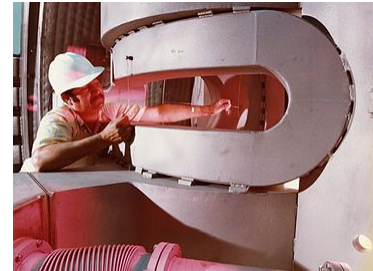
Magnetic mirrors suffered from end losses, requiring high power, complex magnetic designs, such as the baseball coil pictured here.
