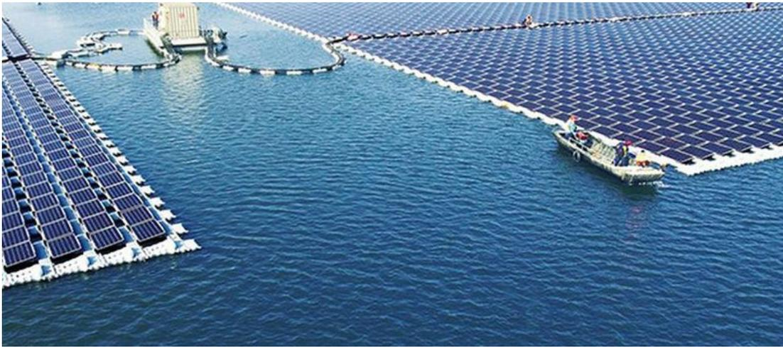
This floating solar array, the largest in the world, produces enough electricity to power 15,000 homes in China. There are 166,000 panels included on the structure.
