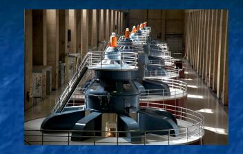
But despite their vastly increased size these still clearly resemble the AC motor from my woodworking tool! Because, at their heart, they DO still have the same components: A stator (likely an electromagnet rather than a permanent magnet) And a rotor (almost certainly an electromagnet) All just waiting for something to turn that rotor!
